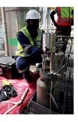
Pressure safety valves installed on industrial plant protect life of employees and avoid damages on equipment in case of excessive pressure. A periodic calibration is one of the most important requirements to ensure that the safety valves will provide this critical protection.
